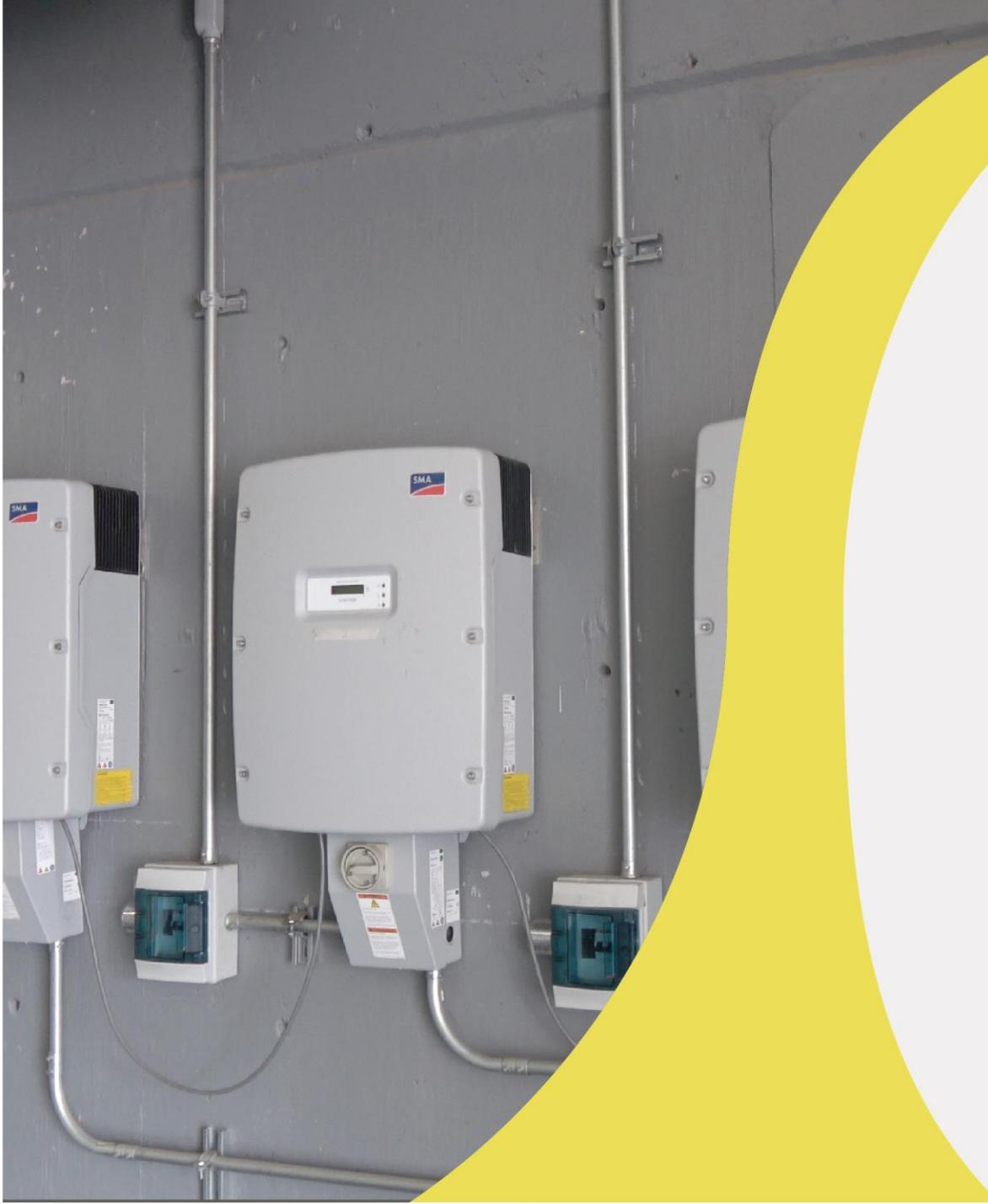
A photograph of several SMA inverters mounted on a grey wall. The inverters are white and grey, with the SMA logo visible. They are connected to a network of metal conduits and wires. A large yellow curved shape is overlaid on the right side of the image, partially obscuring the wall and the inverters.
